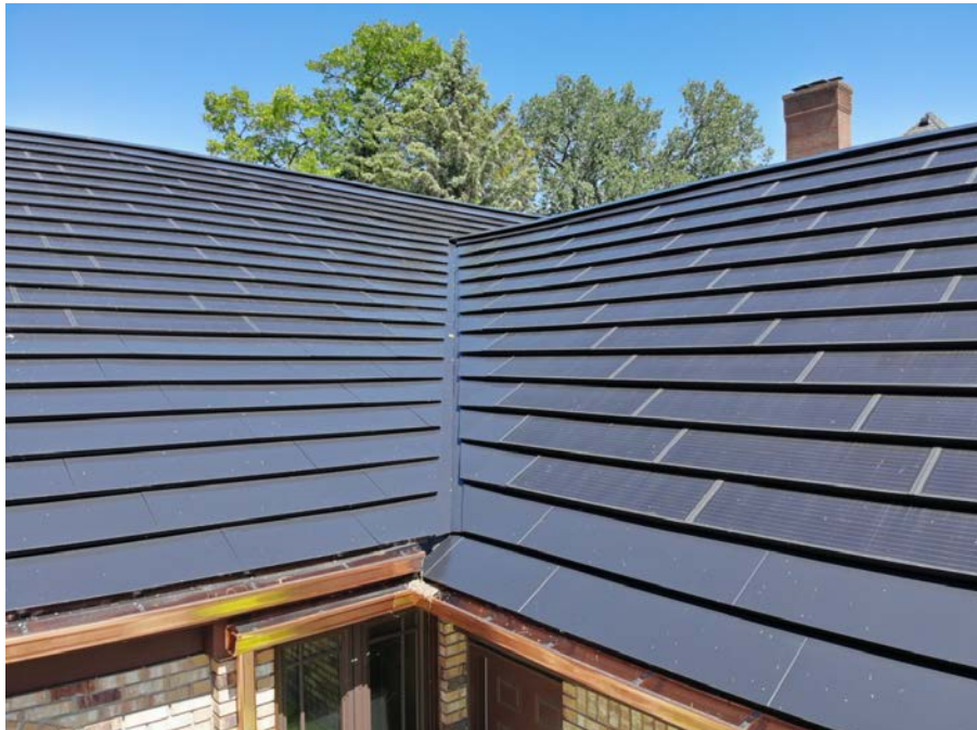
Example above of a Solar Tile installation that has a matching material at the edges that is favored.
